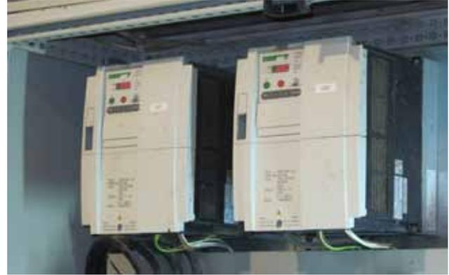
**Figure 11.** Variable speed drive.
