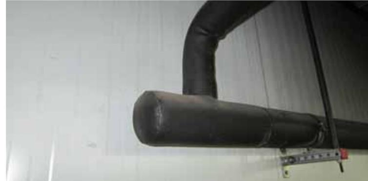
**Figure 12.** Pipe insulation in good conditions.
